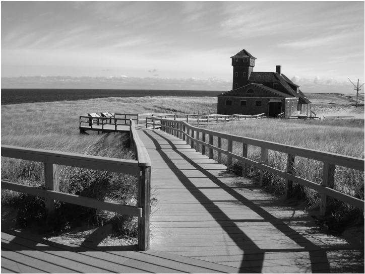
2.13 Boardwalk at Cape Cod National Seashore in Provincetown, Massachusetts
