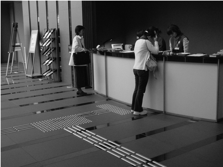
2.5 Tactile floor leading to information desk
