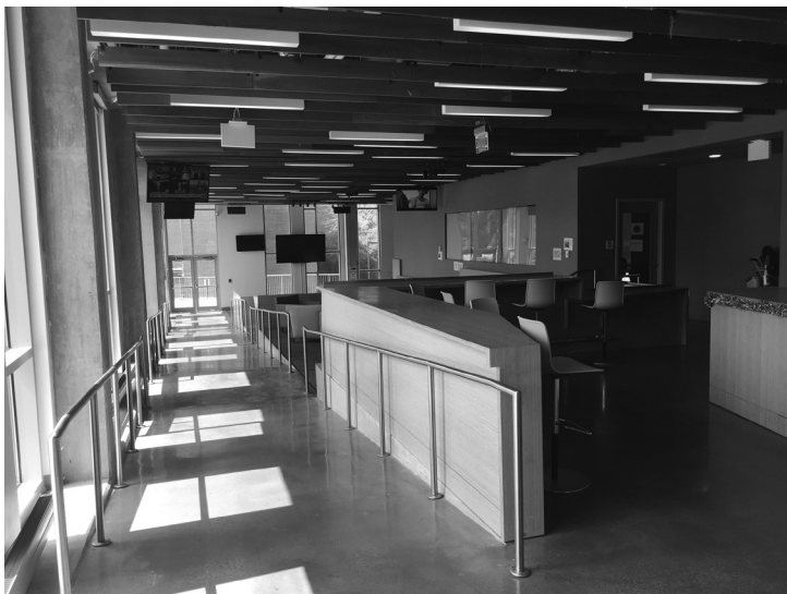
2.21 Suspended acoustic treatment in university presentation space
