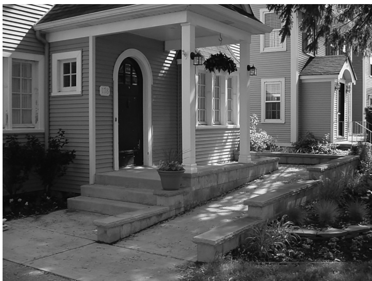
2.15 Ramp to entrance of home
