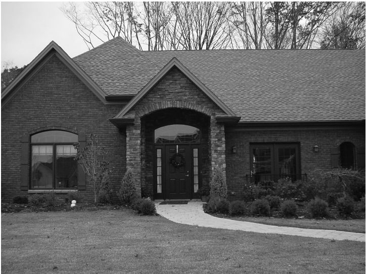
2.16 Sloping residential entry path in home show house by Heartland Homes
