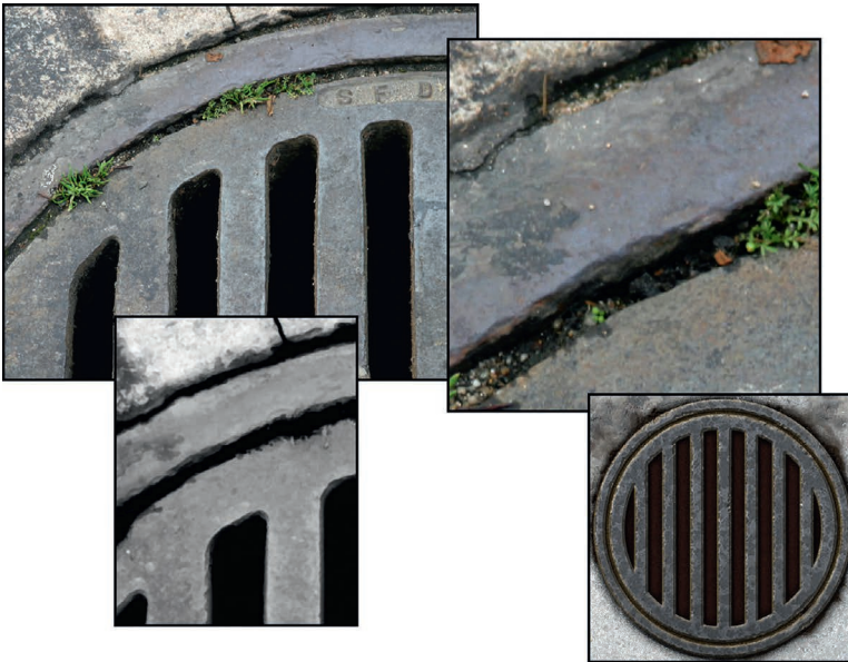
FIG 1.33 This sewer intrigued me: a simple shape of a common item that many might overlook as not worthy of serious attention. Some may have the attitude that it is only a sewer grate, so make it and move on. But a shiny new sewer grate with clean edges would stand out in a grungy urban setting. Look at this sewer grate. It is made of iron and looks solid and heavy. It was probably laid down decades ago and has had thousands of cars drive over it, people walk over it, millions of gallons of rainwater pour through it. On the image at the upper left you can look at the iron and see how it is rusted, but it's so well worn that the rust is polished off in most places. Dirt has built up in the cracks between the grate, the rim, and the concrete. Even little plants have managed to grow. Look at the close-up at the upper right and you can see just how beat-up this iron is and how discolored it has become. At the lower left, I desaturated and cleaned up a portion of the image to see just how the light and shadow are hitting it and to get a feel for the quality of the surface. In this image, you can more clearly see the roughness of the cement and the metal, and although the circular grate looks round from a distance, up close there are no straight edges and smooth curves. All this detail can't be depicted 100% in a game texture, but knowing it's there and understanding what you are seeing will allow you to convey a richer version of the grate as you learn to focus on those details that add realism and character. On the lower right is a texture I did, and you can see that I was able to quickly achieve a mottled and grungy look for the metal and the edges. There are a few places at the top where I started the process of eating away at the concrete and the metal a bit.
